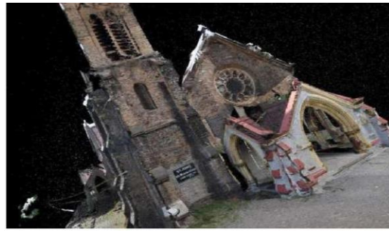
Figure 8: Resultant Point cloud of church after geo-registration
